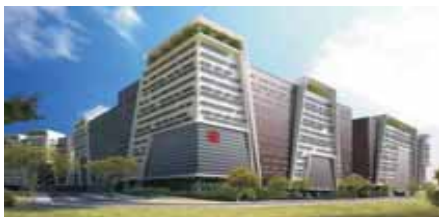
Singapore Industrial Building
